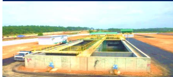
STP WITH CAPACITY 20,000 PE
