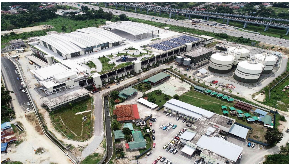
Photo caption: The modern and sophisticated Langat Centralised Sewage Treatment Plant will have the capability to serve up to 920,000 Population Equivalent in Langat catchment area.
