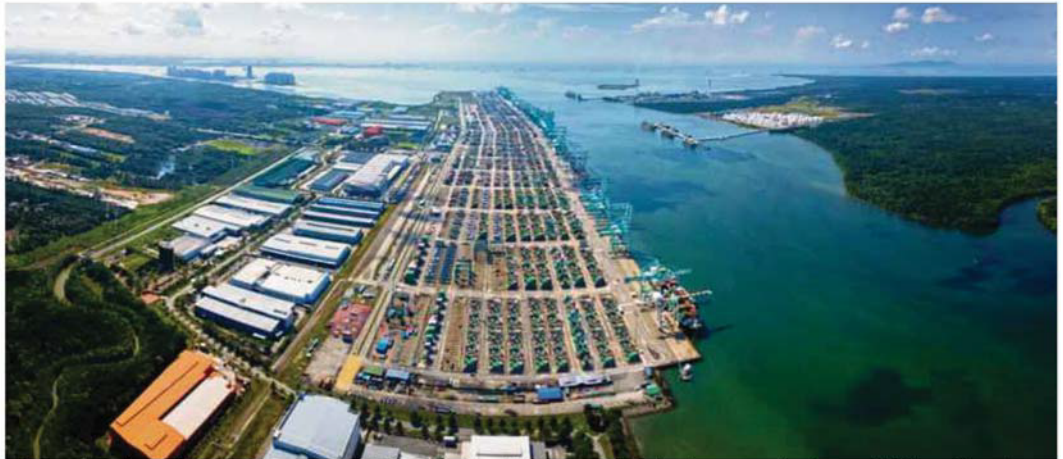
The Port of Tanjung Pelepas in Gelang Patah, which was developed from a green-field site that was previously a small fishing village, is now one of the 20 busiest ports in the world.
