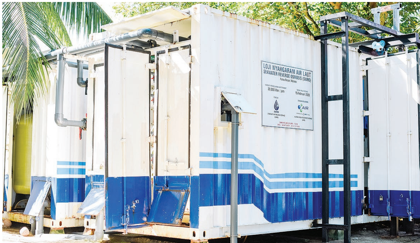
AIR Bhd has also made the SWRO system easy for shipment and site installation by packaging it into containers, creating an opportune environment for its client
