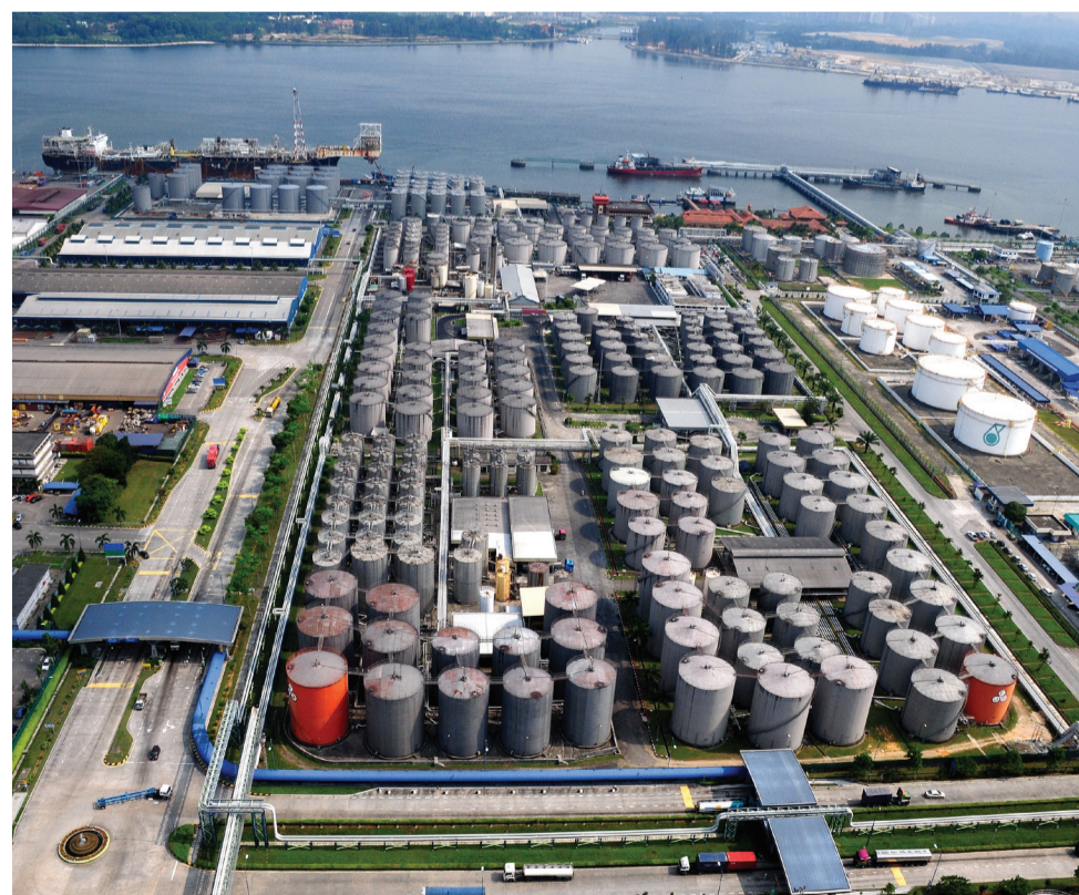
Johor Port's tank farm for edible and non-edible liquid has the capacity of storing 1 million metric tonnes
