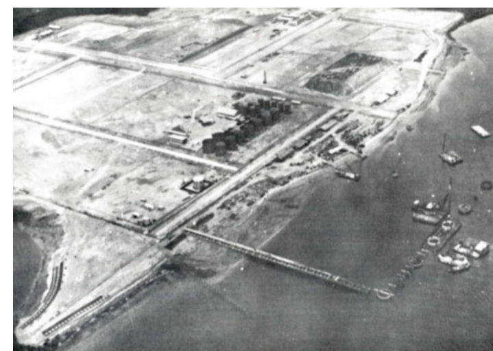
Johor Port under construction
