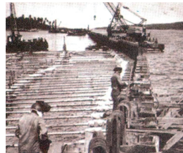
The construction of a wharf
