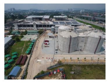
Caption: MMC PLSB is the main contractor for the construction of Langat Centralised Sewage Treatment Plant that has the capacity of 920,000 population equivalent covering a total of 77.6 sq km catchment area starting from Cheras Batu 11 to Kajang. It is designed to achieve the Class 1 water quality, specifically in the ammonia removal. Langat Sewerage Project is one of the initiatives and the main component in the Sewerage Non-River project under the Greater KL programme.
